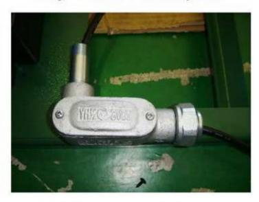
Lock the cover of the steel adapter box.
