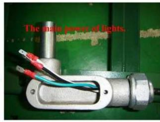
At first take out the cable of light from the steel adapter box.
