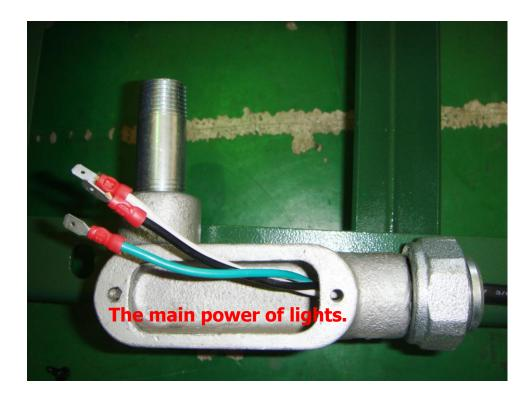
• Then have the cable of the light switch go through the tube into the steel adapter box.
