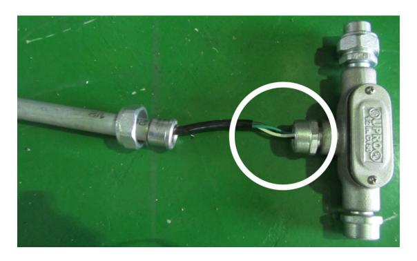
• From the tube number: **5**, take out the cable of the light and install into the steel adapter box.
