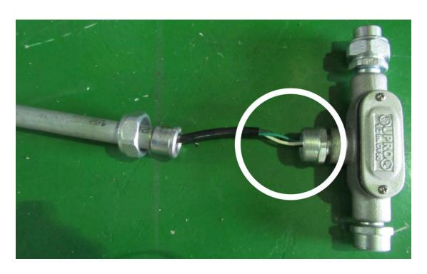
• From the tube number: **2**, take out the cable of the light and install into the steel adapter box.
