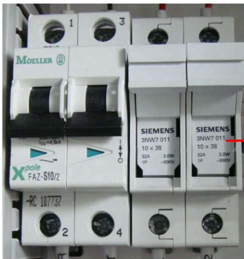
◆ Input relay, fuse bus.
