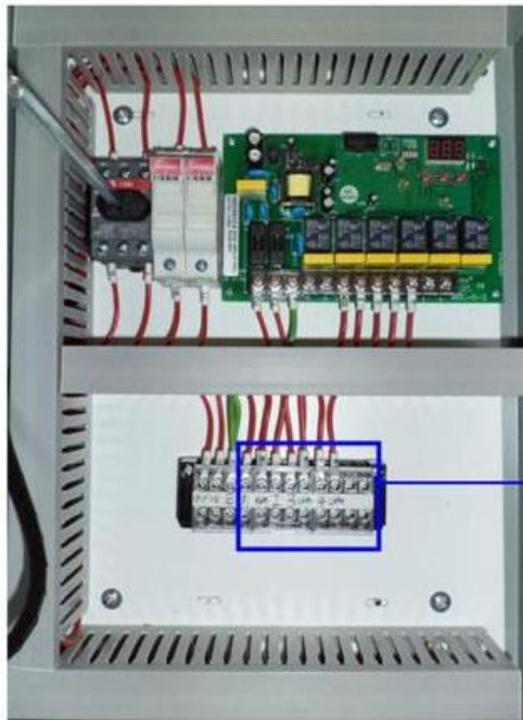
Main Electrical Components for SDC-20-16MDF Pulse Control Box
