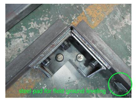
Fasten sleeve anchors (5/8"\*5"L) to field bolted after installations for leveling frame.
