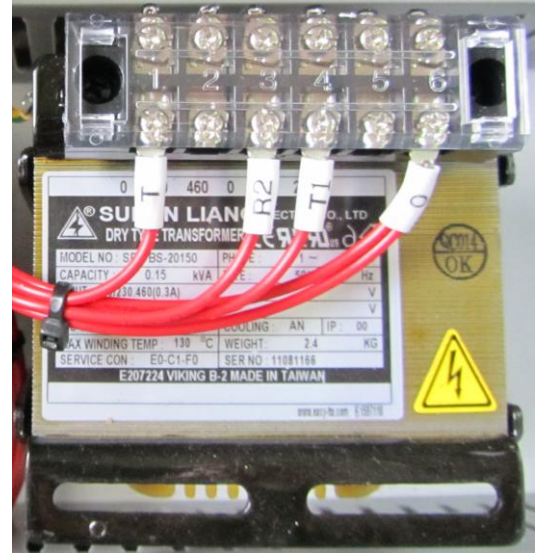
◆ Transformer for 460V.
