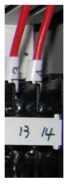
Connect to the right limit switch of the motor 1 for BAY-9.
