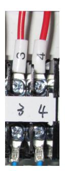
Connect to the left limit switch of the motor 2 for BAY-9.
