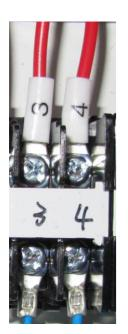
Connect to the left limit switch of the motor 2 for BAY-2.
