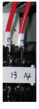
Connect to the right limit switch of the motor 1 for BAY-2.
