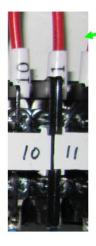
Connect to the left limit switch of the motor 1 for BAY-2.
