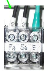
Connect to motor 3 power supply for BAY-2.
