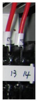
Connect to the right limit switch of the motor 1 for BAY-10.
