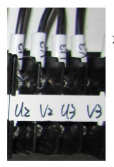
Connect to motor 1 power supply for BAY-10.
