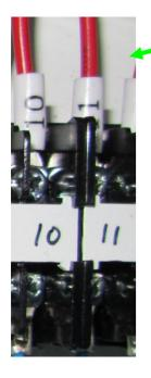
Connect to the left limit switch of the motor 1 for BAY-10.
