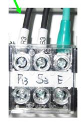
Connect to motor 3 power supply for BAY-10.
