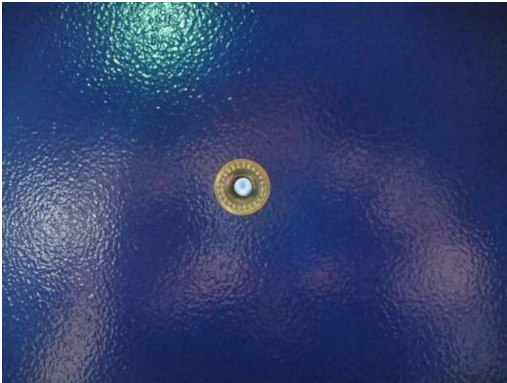
(6) 1/2" inset nuts going through left wall
