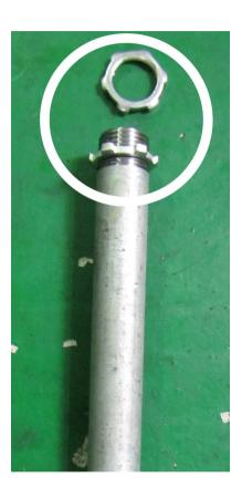
Then, loosen the locknut.
