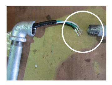
Reach the cable through the number 6 (the tube connecting to the elbow, 90 degree) into the number 7 (the tube)
