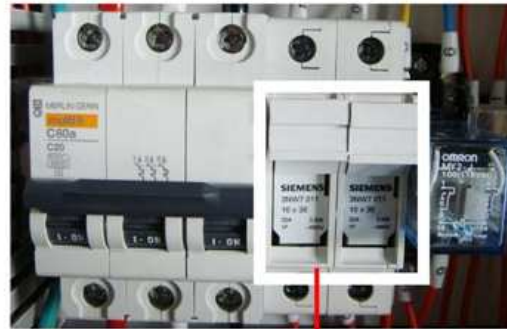
◆ Input relay, fuse bus, phase controller.
