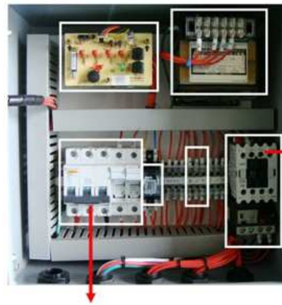
◆ Input relay, fuse bus, phase controller.
