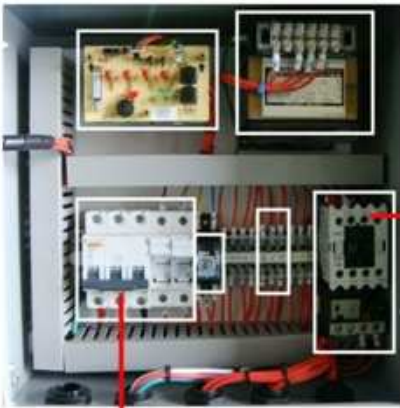
◆ Input relay, fuse bus.
