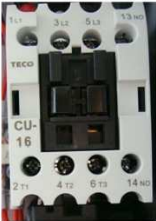
◆ Contactor and thermal relay. (7.5HP-460V)
