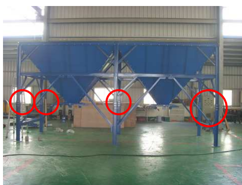
【6】 After insertion, fasten (12) pcs of 1/2''*1-1/4'' Hex Screws, (24) pcs of 1/2''*OD23*2t Flat Washers, (12) pcs of Spring Washers and 1/2'' Hex Nuts at the six locations.
