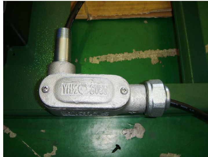
◆ Lock the cover of the steel adapter box.
