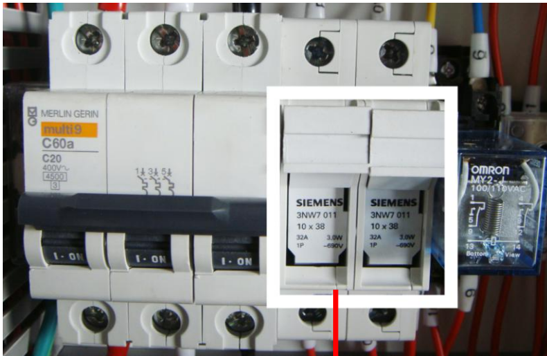
◆ Input relay, fuse bus, phase controller.
